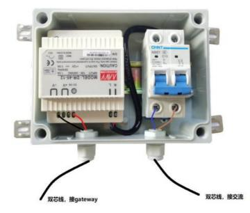
The internal connection scheme of the control box is shown in the diagram above. The AC two-core wire is connected to the lower side of the internal switch; the DC two-core wire connected to the gateway is connected to V+ and V- of the internal power supply.
